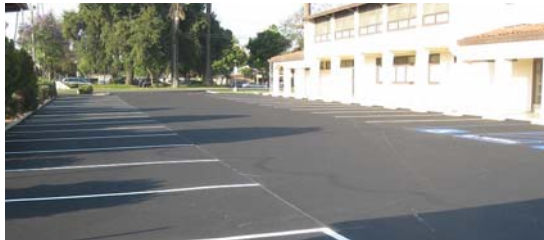
Parking lot was sealed and re-stripped
